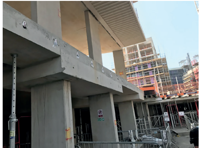
Shear connector headplates are installed
