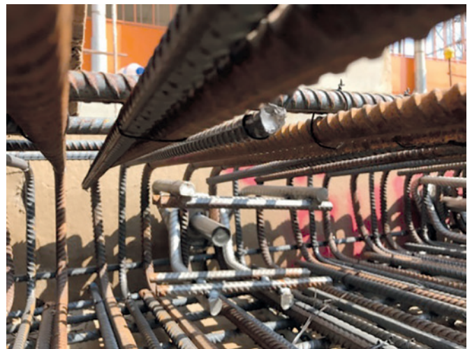
Male part of the shear dowel is connected
