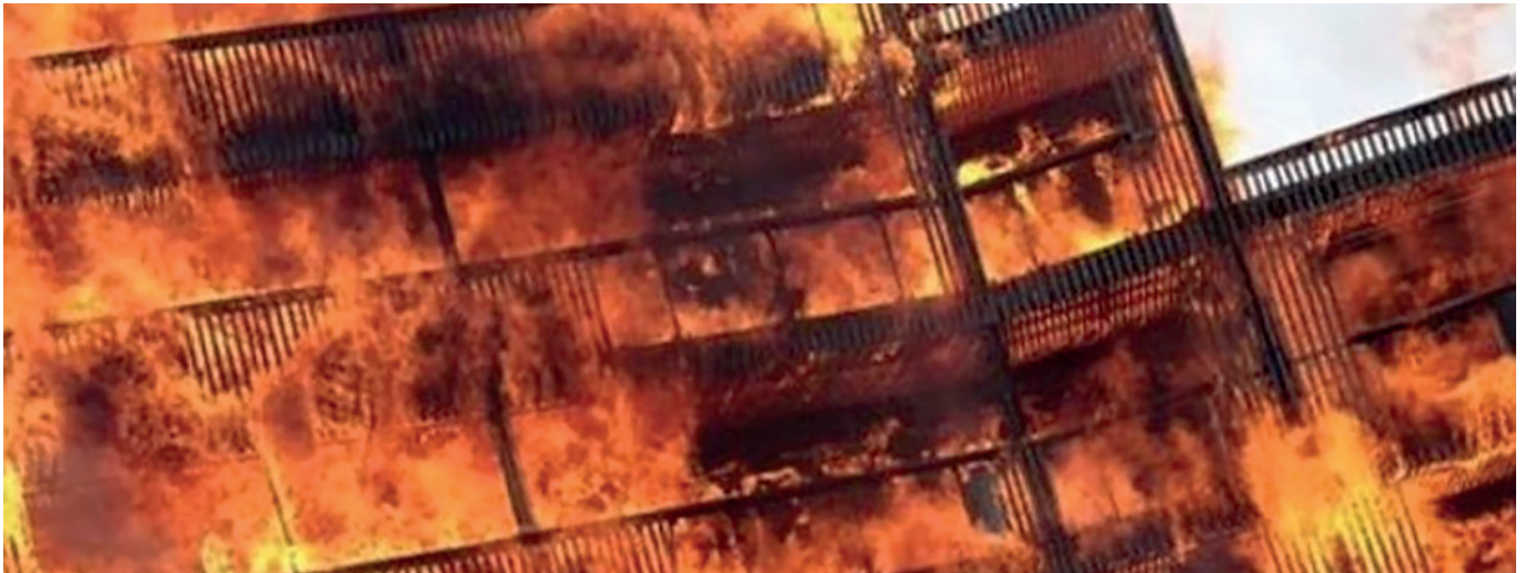
Fire rips through the timber cladding and balconies
